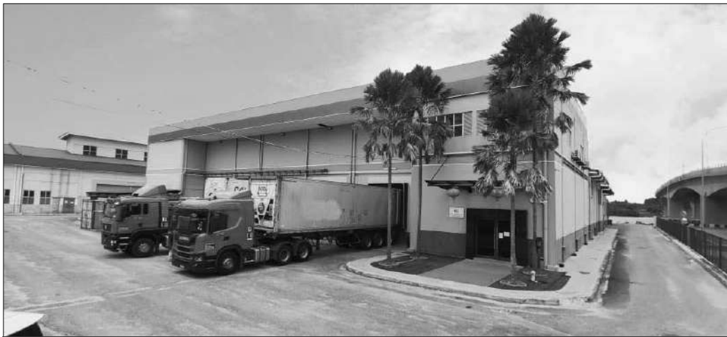
KIFPP Processing Facility
